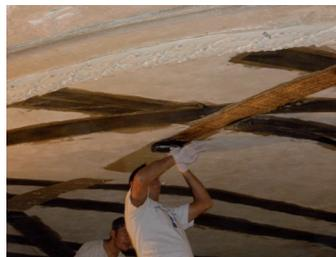
Posa in opera delle fasce in CFRP
